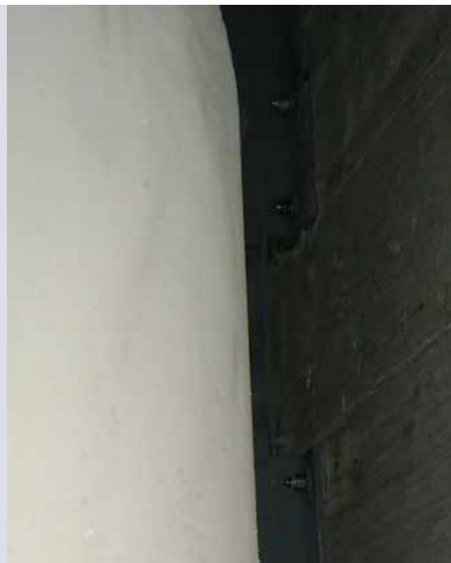
INSTALLATION DE TRANSPORT
